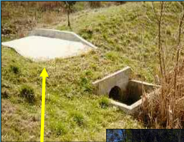
Emergency spillway (often made of stone or grass-lined)
