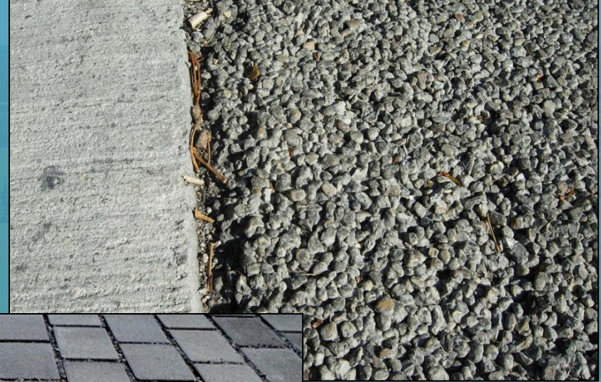
The surface of porous concrete and porous asphalt must be kept clean.
