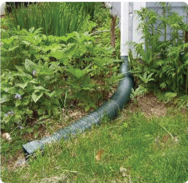
Examples of downspouts for vegetated filter strips
