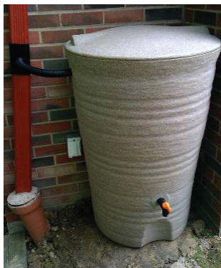
Example of a rain barrel with downspout diverter that directs overflow back to the downspout
