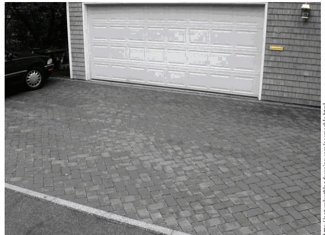
Example of pervious pavers used for residential driveway
