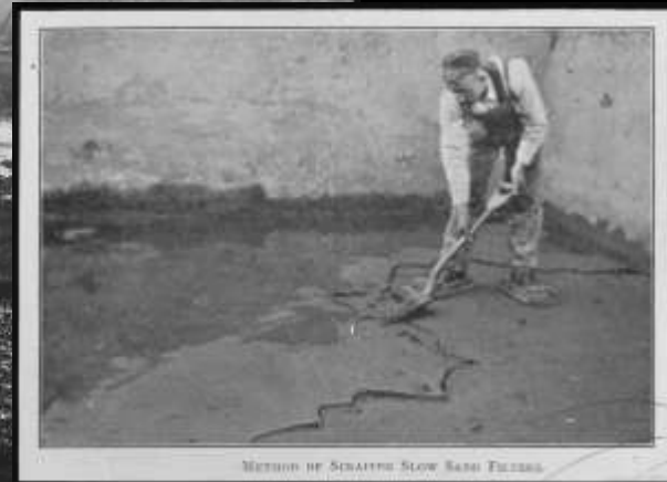
METHOD OF STRIPING SLOW SAND FILTERS
