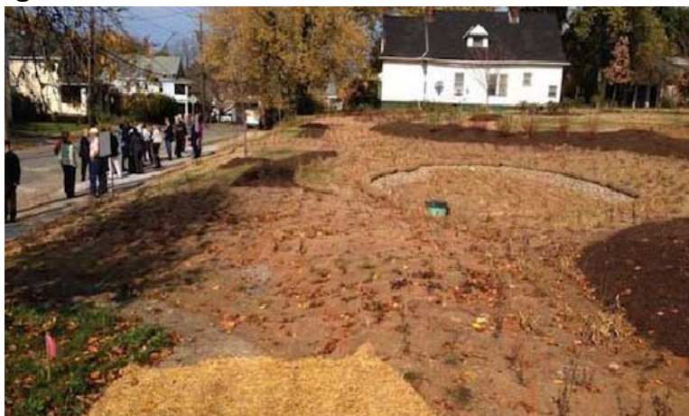
Complete Bioretention Basin on East 78th Street - Slavic Village Demonstration
