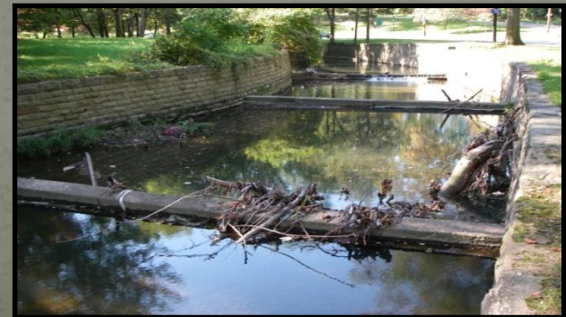
Concrete Check Dams
