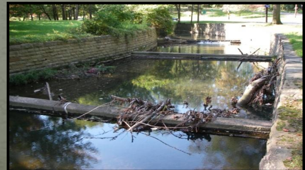
Concrete Check Dams
