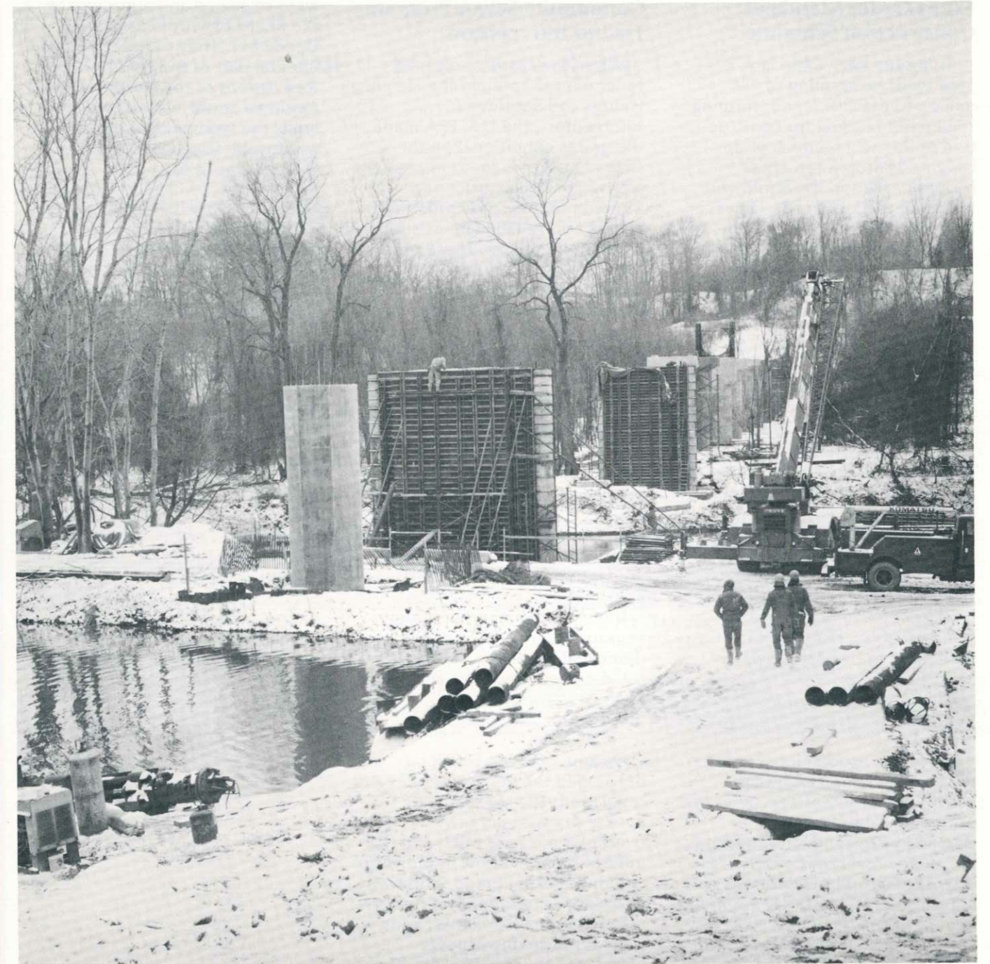
Construction of the Southwest Interceptor continued throughout the winter of 1985. These concrete piers will carry the interceptor across the Cuyahoga River and the Cuyahoga River Valley.
