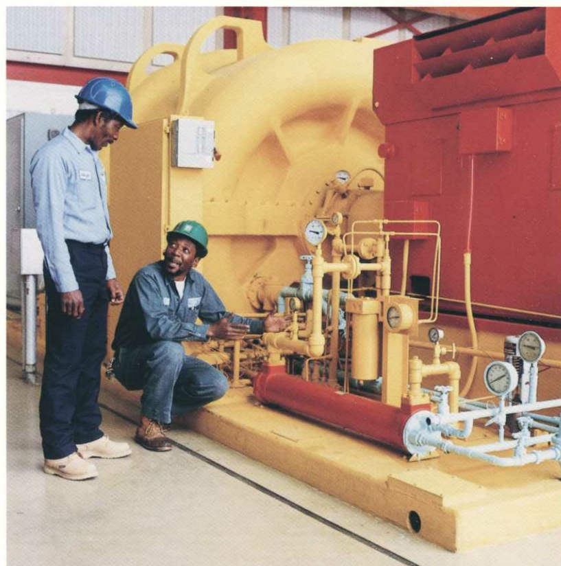
At Southerly, air compressors supply process air to the second stage aeration tanks. Plant Maintenance Mechanic Luther Norman (kneeling) and Operator C2 Bobby Gillespie are assigned to the unit and assure the equipment runs properly.
