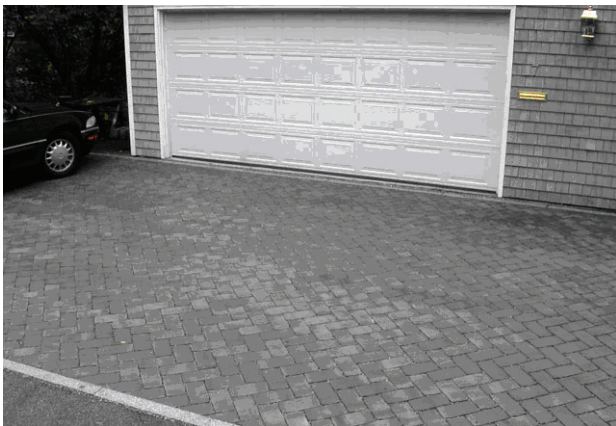
Example of pervious pavers used for residential driveway
