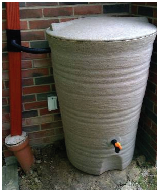
Example of rain barrel with downspout diverter that directs overflow back to the downspout
