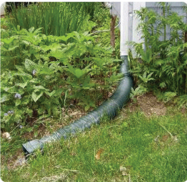
Examples of downspouts for vegetated filter strips
