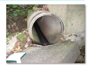
**Problem Summary:** The headwall of the outfall was cracked and had fallen partially northward into the tributary. Additionally, approximately five feet upstream of the outfall opening, the storm sewer pipe completely separated from the remainder of the pipe and flow was discharged into the ground through the crack and not through the opening of the outfall. The concrete headwall and exposed pipes fixed by the City of Mayfield Heights.
