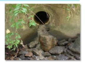
**Problem Summary:** Dry-weather flow with elevated *E. coli* densities was traced to Front Street between 31 Riverside Drive and 87 Front Street. A water main break was also found between 44 and 54 Front Street. The City of Berea is conducting dye tests and working to remediate any problems with improper connections and water leaks in the area.
