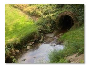
**Problem Summary:** Problem is intermittent. Dry-weather flow was traced to between 14200 Newton Road and 14400 Newton Road. Improper connection between the home at 14223 Newton Road and the storm sewer has already been documented. Other possible improper connections may also be present in area; dye testing by the City of Middleburg Heights should be conducted to determine all sources of sanitary sewage to the storm sewer.
