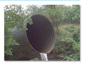
**Problem Summary:** Dry-weather flow with elevated *E. coli* densities was traced to Montrose Avenue and upstream locations. Improper connections were found between St. Mark School and Rectory and the storm sewer. WPC is working with St. Mark to remediate the problems.
