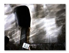
**Problem Summary:** Flow with elevated *E. coli* densities was traced along Euclid Avenue to Grand Boulevard. A video inspection of the area indicated improper connections between the apartment buildings located at 20200 and 20240 Grand Boulevard and the storm sewer. Recommend that the City of Euclid conduct dye testing to verify improper connections.
