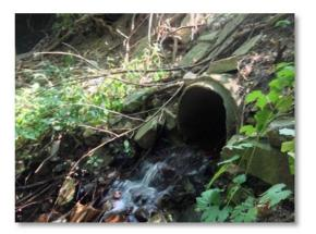
**Problem Summary:** A blockage within the sanitary sewer at Broadview Road and Broadrock Court was remediated; however, during the Sewer District's September 22, 2015, re-inspection following corrective action by the City/CCDPW, the Sewer District observed that the hole in the sanitary sewer was allowing sewage to exit the sanitary sewer during high flows/surcharging and enter the adjacent storm sewer.
