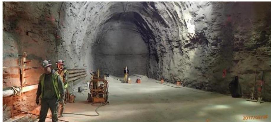
Figure 9 Dugway Storage Tunnel under construction
