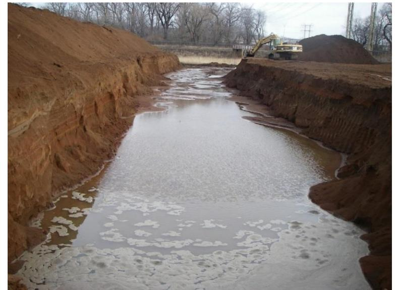
**Figure 3** Ash Lagoon at Southerly Wastewater Treatment Plant. The Beneficial reuse program will result in diverting nearly all biosolid incinerator ash from landfill.
