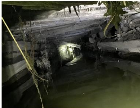
Figure 6: BA00013 Deteriorated Timber Section
