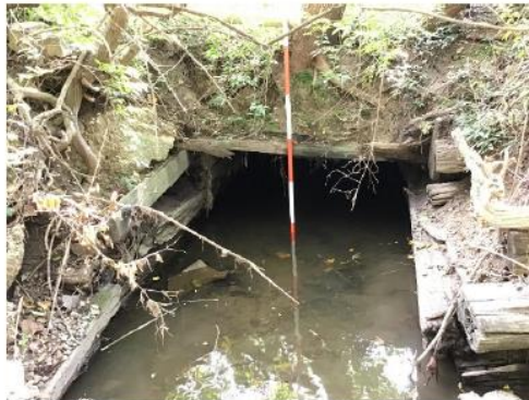
Figure 7: BA00013 Failing Timber at Outfall Section
