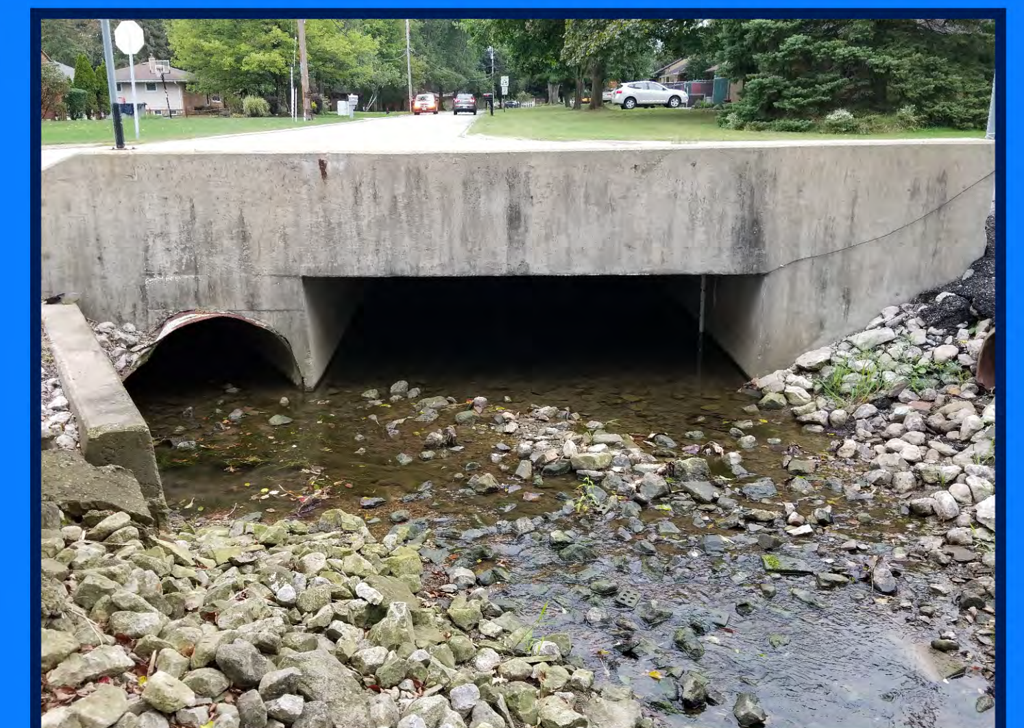
Existing storm sewers that convey flow from Stream CC00184 and local storm sewers, under Wallings Road, to the downstream sections of Chippewa Creek.
