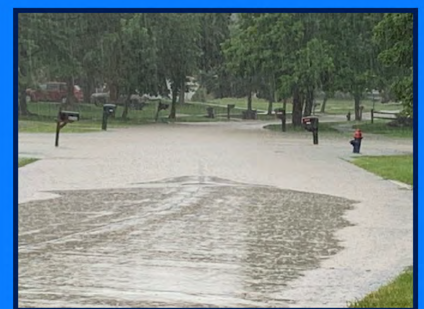
Flooding on West Ridge (July 2019)
