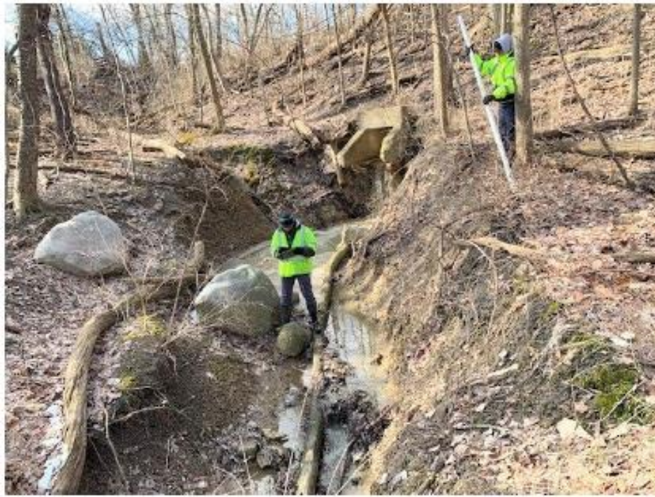
Brecksville Road culvert outlet Contributes about 18 tons sediment/yr (6%)
