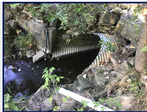
Existing Culverted Stream Outlet at Stream CC00184
