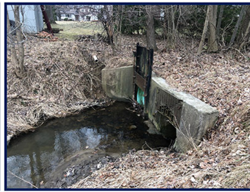
Existing Basin Outlet Structure
