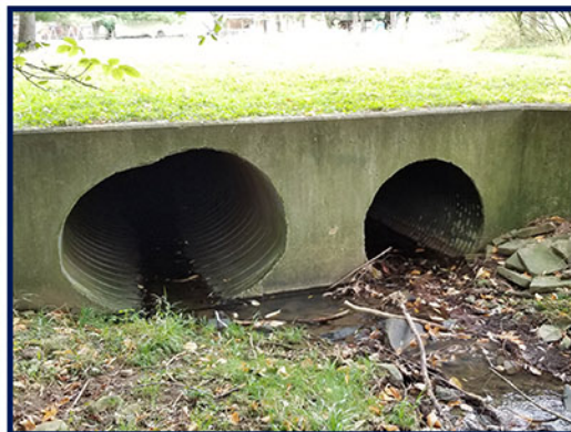
Existing Stream Outlet at Culverted Stream CC00183
