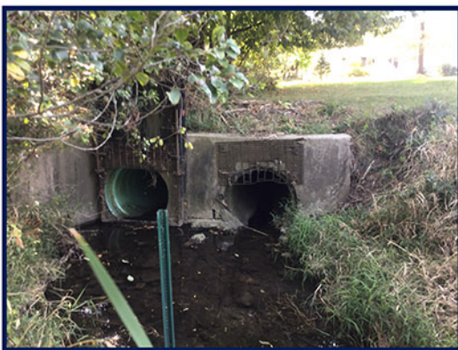
Existing Culverted Stream Inlet at Basin CC00231
