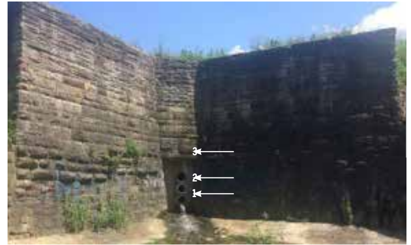
Civil Works Administration (CWA) masonry, 1934
