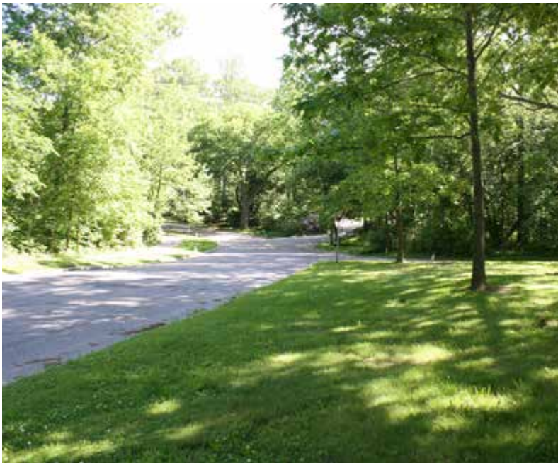
The existing condition of the entrance drive to Horseshoe Lake Park
