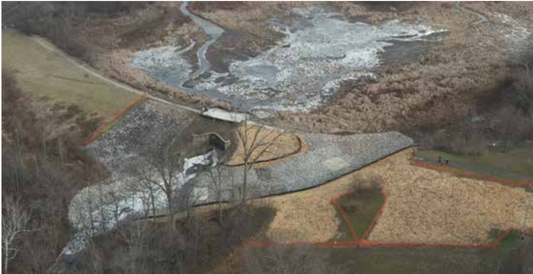
Temporary breach of the Horseshoe Lake Dam.
