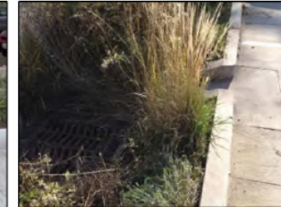
Weeds and untrimmed plantings prevent stormwater runoff from entering the bioretention area from the curb cut. Credit: Northeast Ohio Regional Sewer District
