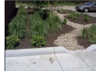
Planted bioretention area with sidewalk curb cut in foreground. Stormwater runoff is conveyed through gravel to shallow depression of bioretention area. Credit: Northeast Ohio Regional Sewer District
