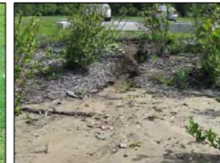
Erosion of side slopes and subsequent sediment accumulation within bioretention area and contribute to clogging issues. Credit: Summit Soil & Water Conservation District
