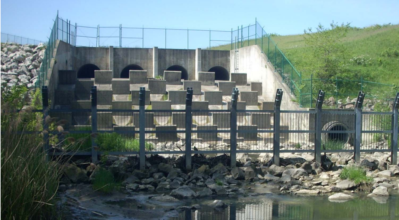
Figure 2. Above photo is the discharge of Abram Creek culvert from the airport expansion.
