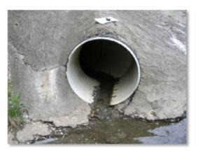
**Problem Summary:** During a previous investigation in 2010, dry weather flow with elevated *E. coli* densities was traced to between 4931 Henry Street and the intersection of Henry Street and Crest Avenue. Improper connections between homes and the storm sewer may be present. Dye testing should be conducted to determine all sources of sanitary sewage to the storm sewer in the area.
