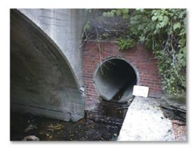
**Problem Summary:** Dry weather flow was traced to Manorford Drive and Alyesworth Drive. Improper connections between homes and storm sewer may be present. Dye testing should be conducted to determine all sources of sanitary sewage to the storm sewer.
