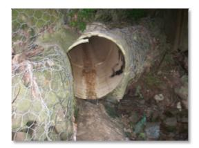
**Problem Summary:** Dry weather flow was traced to Clearview Drive between Lucy Drive and Eureka Parkway in Parma Heights. Improper connections between homes and storm sewer may be present. Dye testing should be conducted to determine all sources of sanitary sewage to the storm sewer.
