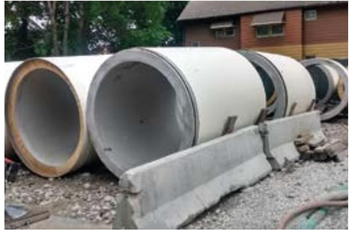
*Concrete pipe awaits descent to line the microtunnel.*
