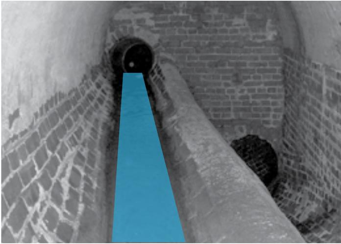
Normal “dry-weather” flow travels to the wastewater treatment plant
