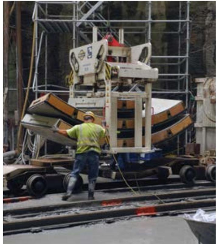
*Pieces of tunnel lining are placed on the segment car.*
