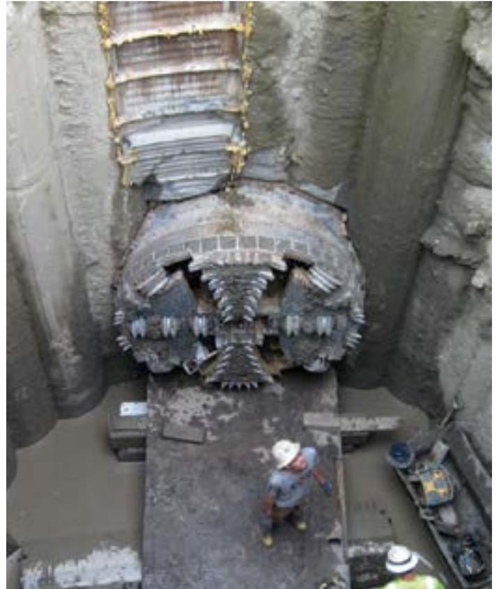
*The MTBM cutter head breaks through the destination shaft wall, completing the DWIRS excavation.*
