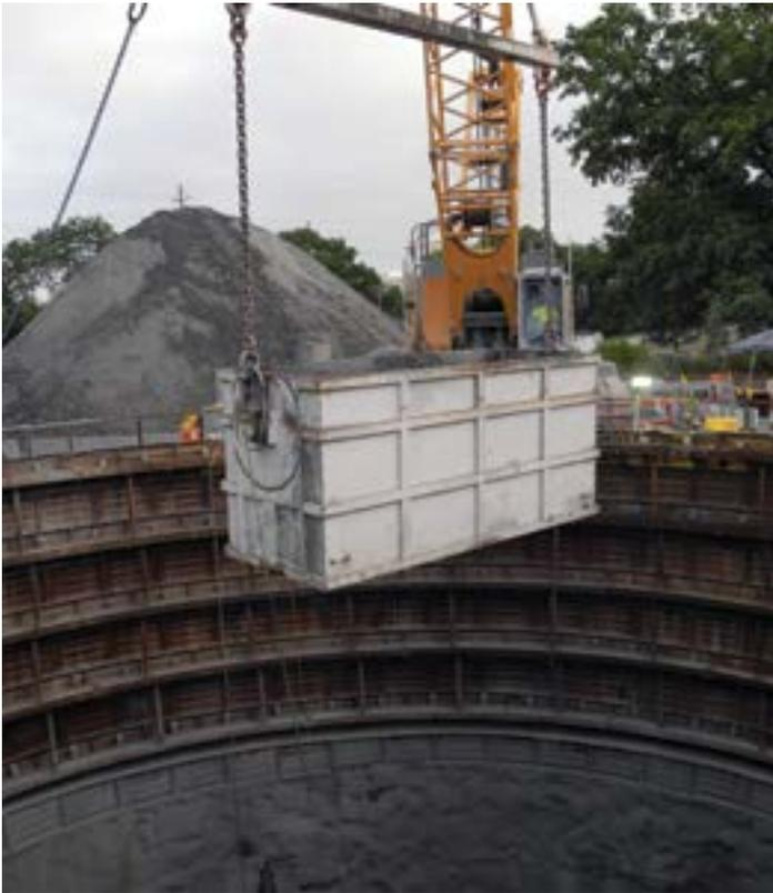
*A crane unloads a muck box full of excavated shale.*
