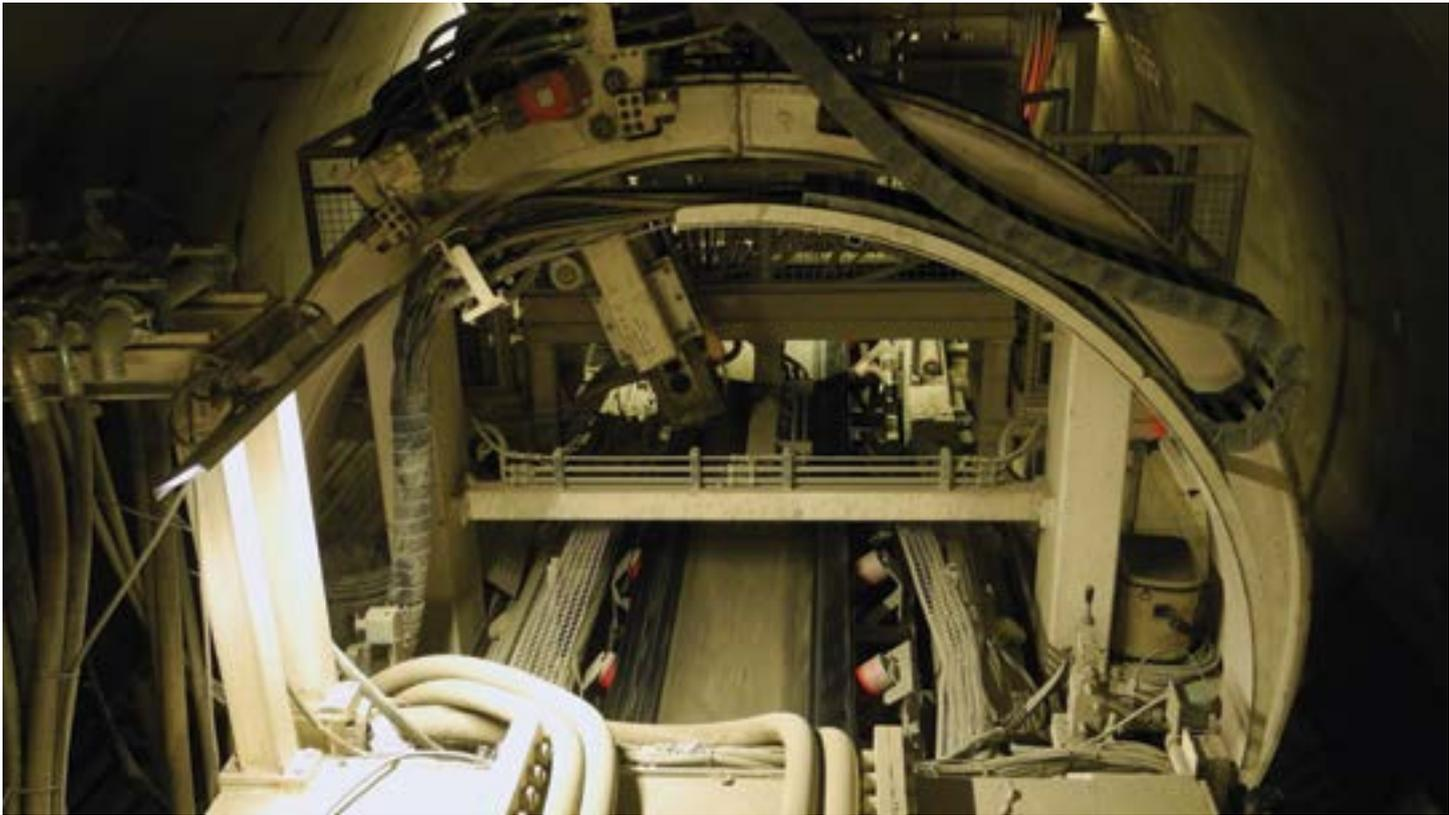
*Overhead view of the front of the TBM. The conveyor belt (bottom center) carries excavated shale from the cutter head to the muck cars.*
