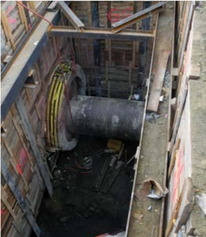
*This old brick sewer has been cut so that it can tie into the new diversion structure for WST (*see next page*). Until then, a temporary steel pipe maintains flow to the Westerly treatment plant.*
