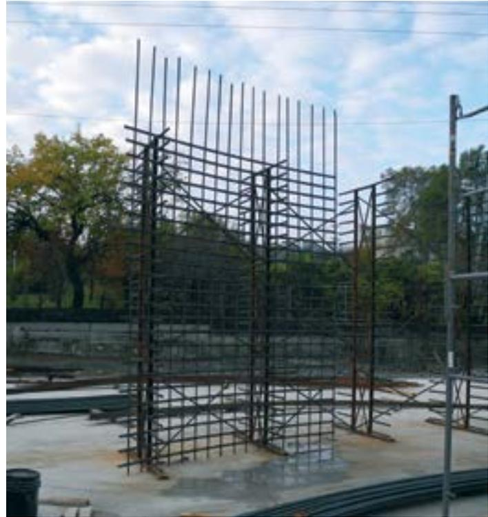
Rebar cage used to make the slurry wall lining
