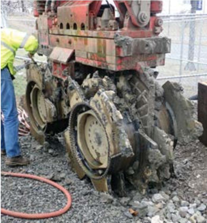
Hydromill used to excavate the WST slurry wall
