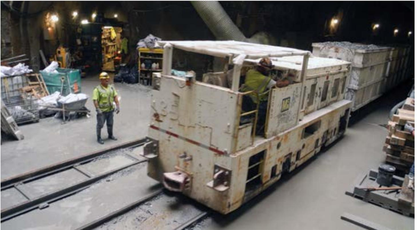
*The locomotive and its muck cars full of excavated shale return to the shaft.*
