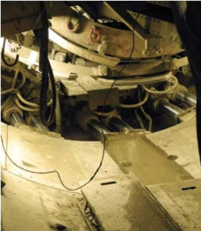
*The TBM pushes itself forward on hydraulic jacks.*
