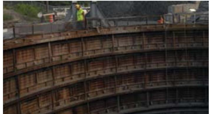
Steel liner plate shaft for the Doan Valley Tunnel
