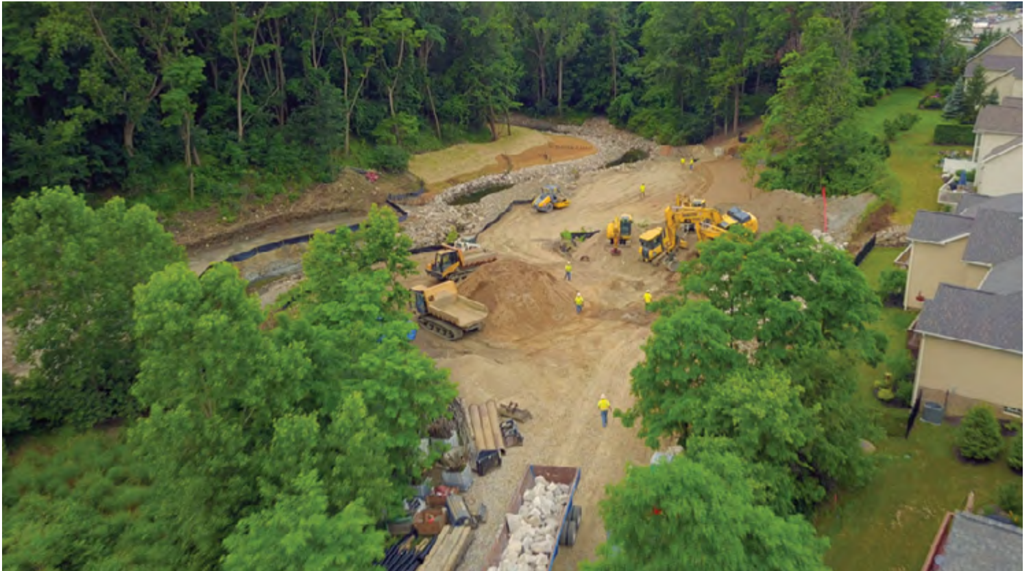
The stream was moved away from the steep eroding banks, and given plenty of floodplain.
