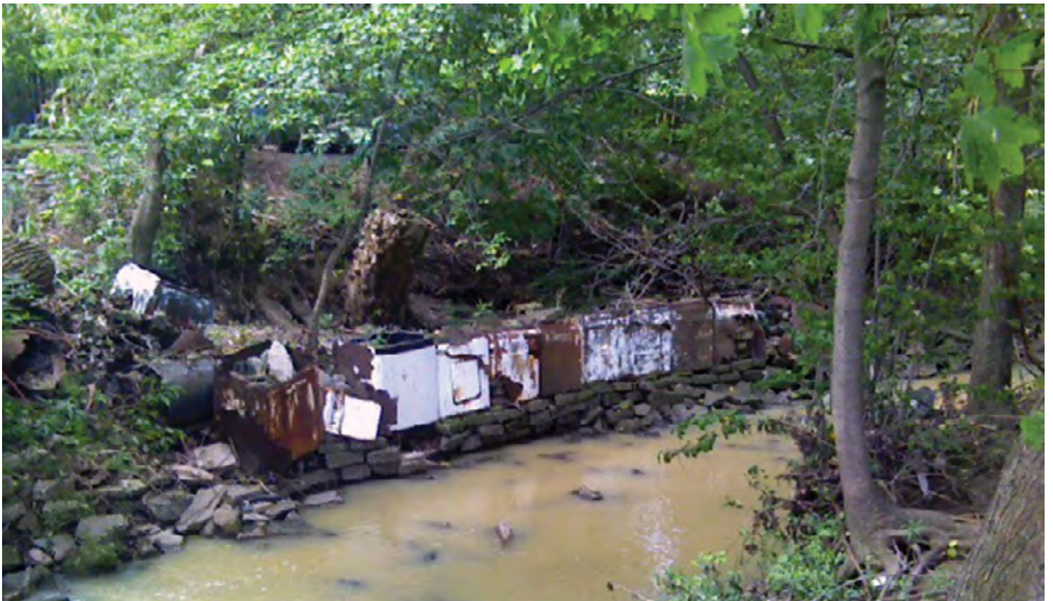
A barricade of used appliances forestalls erosion along Stickney Creek.
