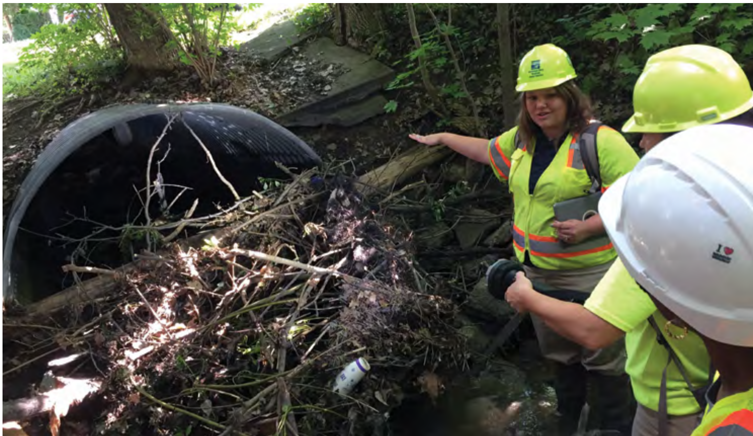
Stormwater Inspector Christina Silea and SWIM co-workers encounter a culvert blocked by debris.
