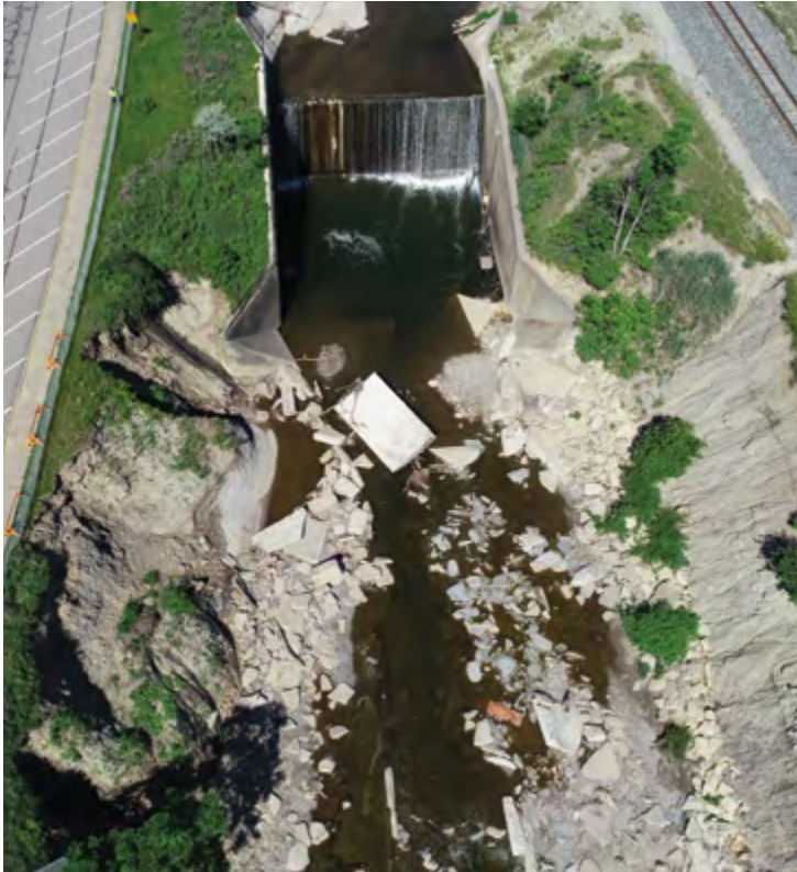
A failing concrete drop structure threatened a nearby road and railway. The Big Creek Stabilization Project included a rock cascade on top of the existing spillway. Now, Big Creek's flows are more natural, allowing fish to navigate the area that had previously been cut off by the spillway.
