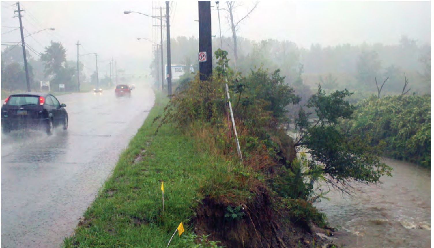
Streambank erosion on Mill Creek creeps towards Warner Road in Garfield Heights.
