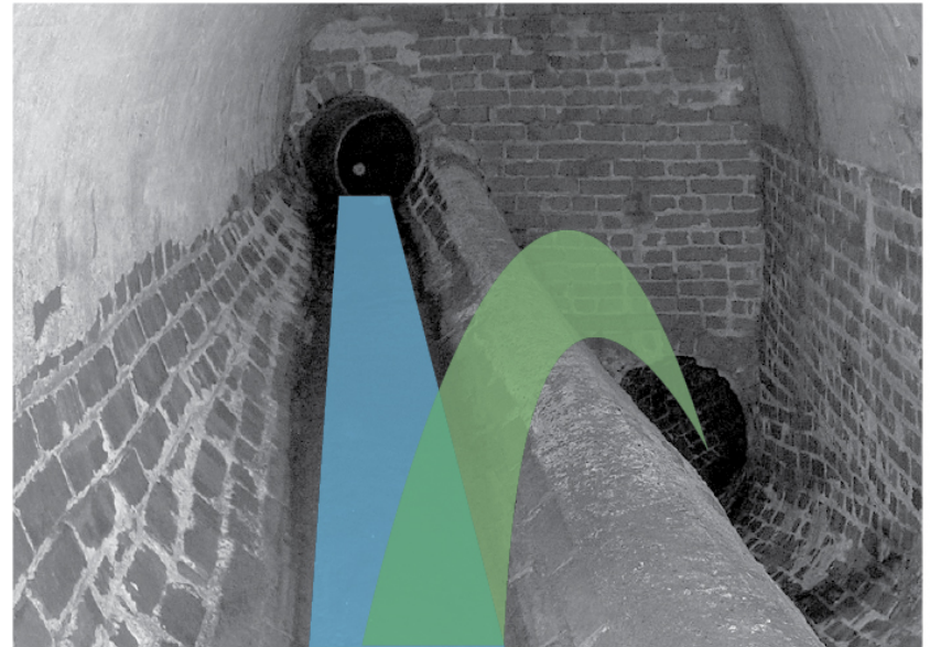
When it rains, a mix of stormwater and wastewater spills over the weir and discharges into the environment, untreated.
