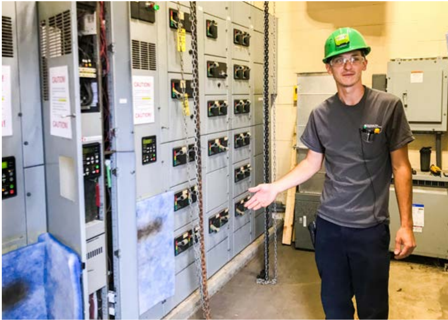
Fowler explains the variable frequency drive: it controls the speed of the motor on a grit pump.
