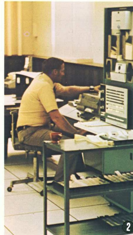
① Sewer flow is ② monitored by a central computer ③ via telemetry and telephony lines.
