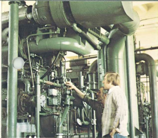
Aeration tank blower motors
