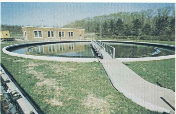
Final settling tank
