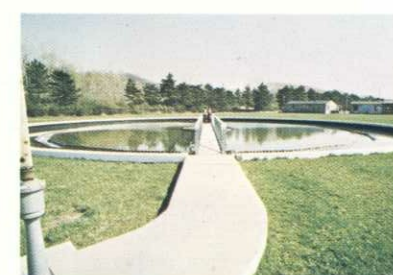
Final settling tank
