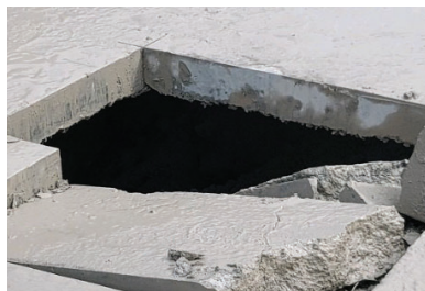
Saw cut and removal of concrete walkway over Horseshoe Lake spillway to investigate detected voids within the dam and spillway structure, July 2021
