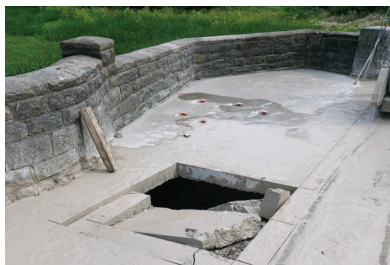
Saw cut and removal of concrete walkway over Horseshoe Lake spillway to investigate detected voids within the dam and spillway structure, July 2021
