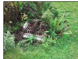
Stormwater flow will be blocked by the dead vegetation on the outlet catch basin grate. Credit: Chagrin River Watershed Partners
