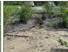
Erosion of side slopes and subsequent sediment accumulation within bioretention area and contribute to clogging issues. Credit: Summit Soil & Water Conservation District
