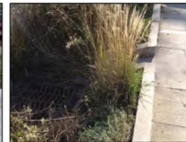
Weeds and untrimmed plantings prevent stormwater runoff from entering the bioretention area from the curb cut. Credit: Northeast Ohio Regional Sewer District
