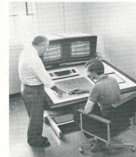
Using the District's new digitized mapping workstation, Sewer Control Systems Superintendent Tony Jordon (standing) and Engineering Aide Jeffrey Pokorny locate the interceptor sewers for input into the computer.
