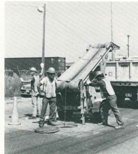
Field Technician Matthew Hill directs traffic while Field Technicians Phillip Caruso (center) and Michael Pelly operate a bucket machine as it cleans a manhole leading to an interceptor sewer.
