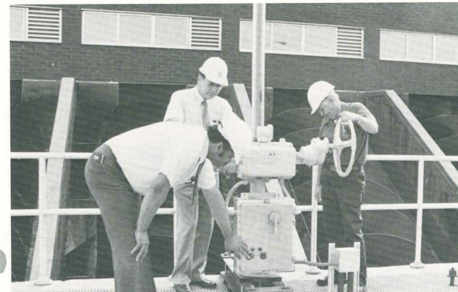
Herman Bishop, assistant superintendent of operations at Easterly, checks the mechanism for the control gate at the plant's screw pump installation with Alex Balazs, superintendent, (center) and Ronald McCune (right), assistant superintendent of maintenance.
