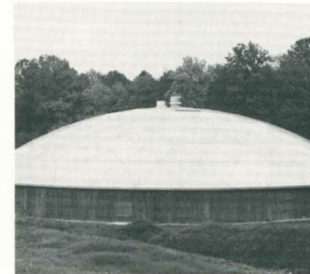
A view of the new aluminum dome covering the Bonnieview stormwater holding tank.
