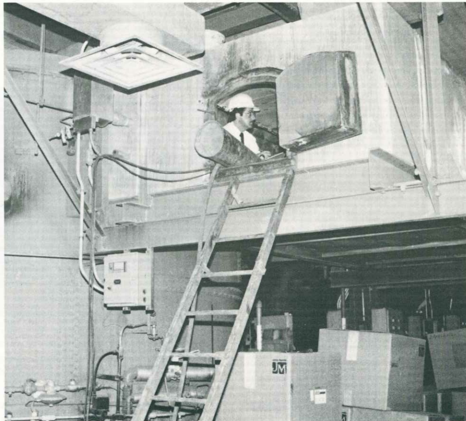
Robert Dominak, project manager, inspects installation of the new lining system for the ductwork of one of Southerly's sludge burning incinerators.
