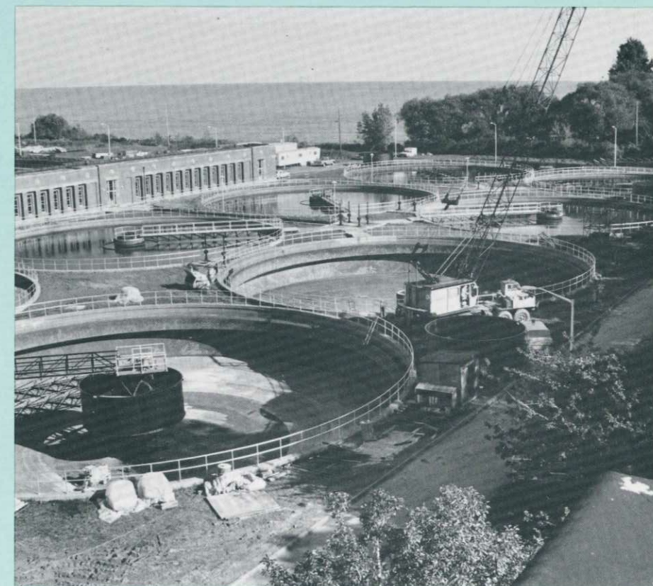
At Easterly, all mechanical equipment in the final clarifier tanks is being replaced.
