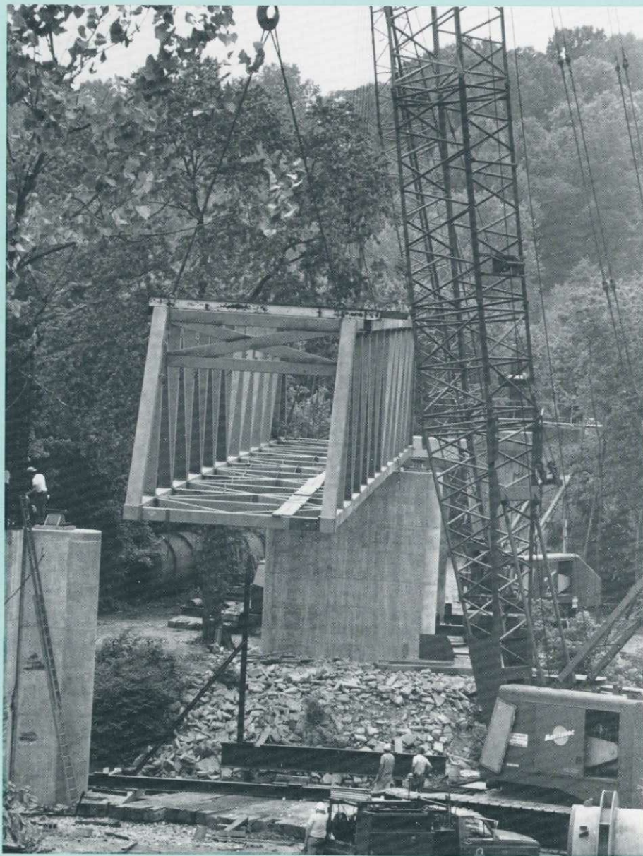
A section of steel truss bridge is lifted by a crane for placement on the concrete piers that will support it. This structure carries the Southwest Interceptor sewer 1,150 feet across the Cuyahoga River and the Cuyahoga River Valley.
