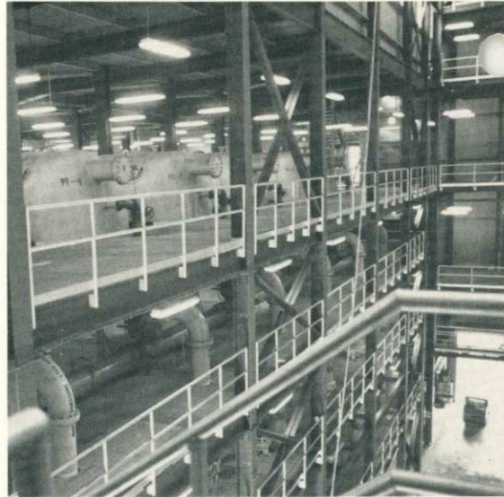
Pictured are some of Westerly's 14 pressure filters that were clogging until the change was made from lime to ferric chloride.
