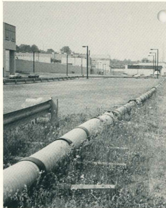
The temporary ash line leads out of the basement of the Incinerator Building at Southerly. It is laid on railroad ties and secured in place with rubber straps.
