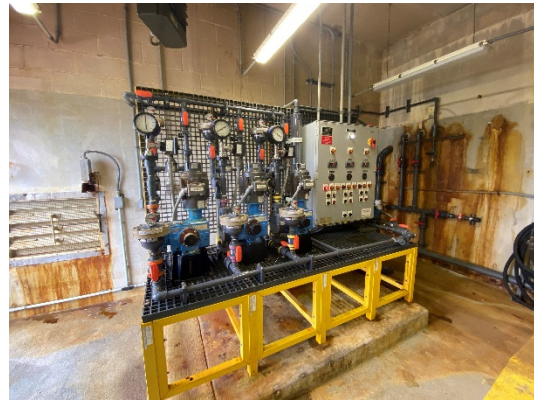
Southerly Ferric Chloride Pumps allow for accurate dosing
