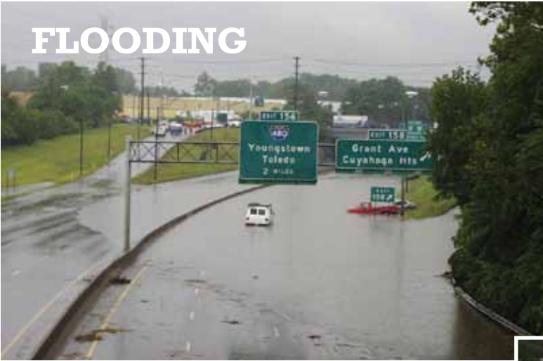
Flooding of Interstate 77 in Cuyahoga Heights
