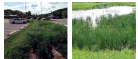
Above are some examples of stormwater control measures more common to non-residential properties.
