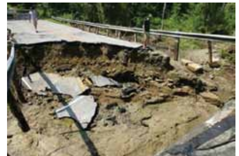
Streambank erosion alongside homes near Chippewa Creek in Brecksville
