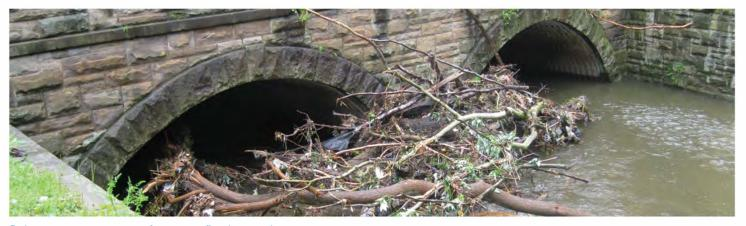
Debris is a common cause of upstream flooding in urban streams.
