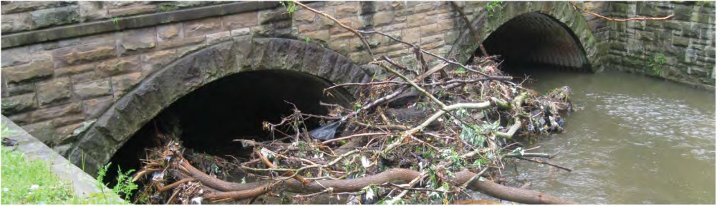
Debris is a common cause of upstream flooding in urban streams.
