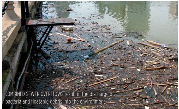
This is a COMBINED SEWER OVERFLOW. This outfall on was at the top of Mill Creek Falls and would discharge during very heavy rains.
