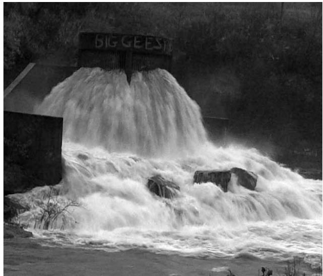
During heavy rains, a combination of rainwater and wastewater—“CSO”—discharges to the environment.
