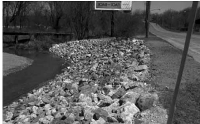
“Before” and “after” photos of an emergency bank stabilization along Mill Creek and Warner Road, a 2013 stormwater construction project.
