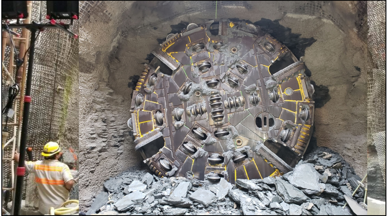
This is hole through or hole out in Doan Valley Tunnel
